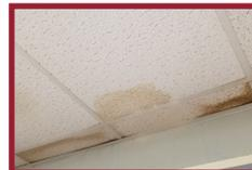
Leaks need to be identified and repaired; stained ceiling tiles need to be replaced once repairs are completed.
