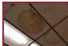
Ceiling tiles were stained and multiple tiles were missing.
