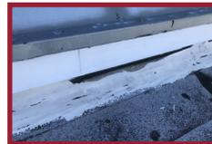
The exterior of the relocatables have issues with damaged skirting and deteriorated sealants.
