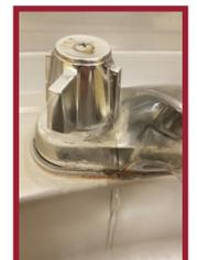
Leaking or loose plumbing fixtures or related components needed to be repaired.
