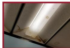
Stained ceiling tiles were observed in all inspected buildings and need to be replaced once the cause is identified and repaired.
