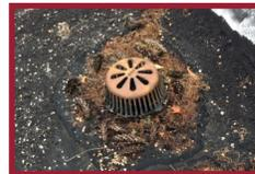
Many roof drains were full of debris and require more frequent inspections and cleanings to ensure proper operation.
