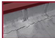
Additional repairs and sealing were needed at many schools where Flashing & Gravel Stops were an issue.
