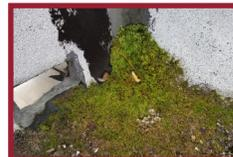
Roofs were observed with vegetation and failing seams.
