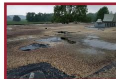
Both inspected schools received a failing rating for their roofs; the roofs were deteriorated with areas of vegetation, blisters, splits and other deficiencies.
