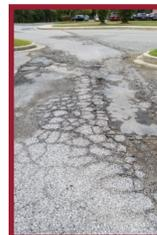
The driveways and parking lots were observed cracking and deteriorated at half of the schools inspected.
