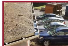
Many gutters were blocked with debris and some gutters and downspouts were damaged.
