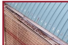
Many gutters and downspouts were damaged, disconnected, leaking or filled with debris.
