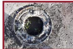
Routine inspections and cleanings were needed at the roof drains to address multiple issues from excessive gravel and debris to cracks and blistering of the membranes.
