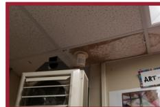
Stained ceiling tiles should be replaced once the cause is identified and repaired.
