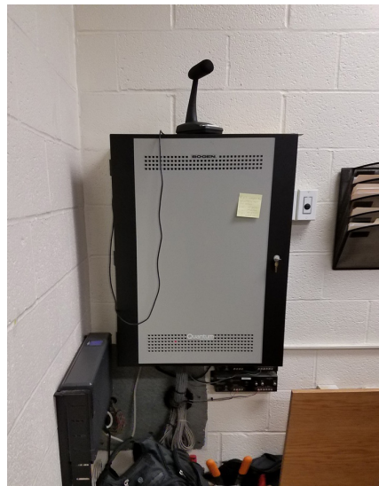
Existing Photo: Public address system control panel.
