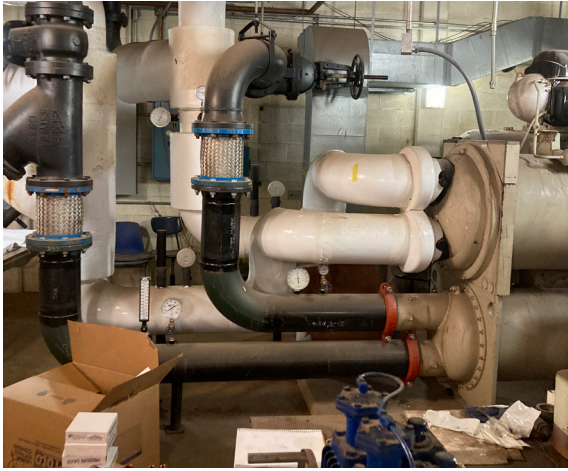
Existing Photos: Existing Chiller (Boiler Room, Building B)
