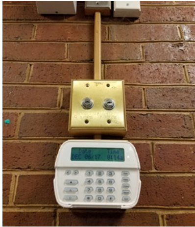
Existing Photo: Intrusion detection system keypad.
