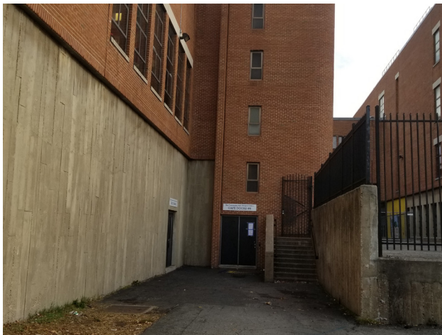
Building B: Showing concrete base with masonry above.
