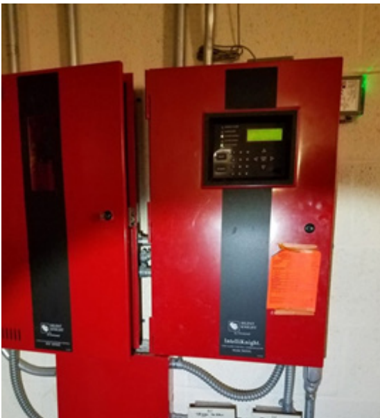
Existing Photo: Fire alarm control panel for cafeteria and auditorium.
