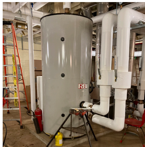
Existing Photo: In-progress HW Heater Replacement
