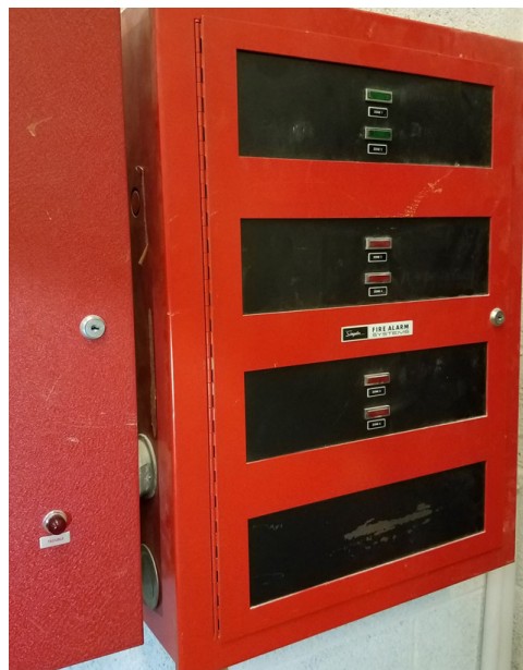
Existing Photo: Fire alarm control panel for most of the building.
