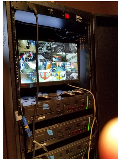
Existing Photo: CCTV system rack.
