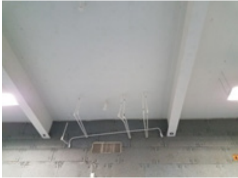
Existing Photo: Hanging conduit in Gymnasium.
