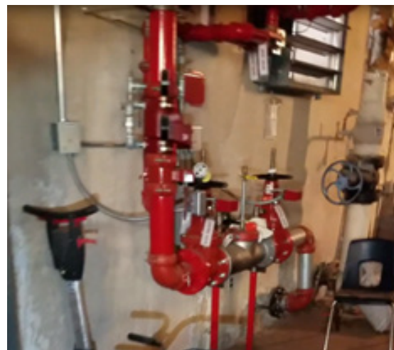
Existing Photo: Incoming fire service with backflow preventer.
