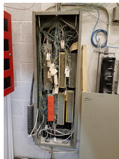
Existing Photo: Telephone punch blocks.
