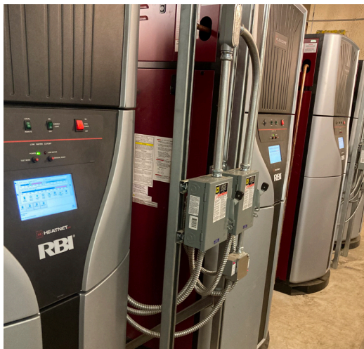
Existing Photo: In-Progress HW Heater Replacement
