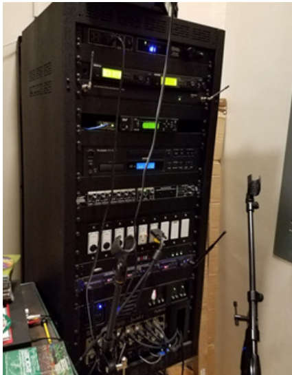
Existing Photo: Auditorium sound system rack.
