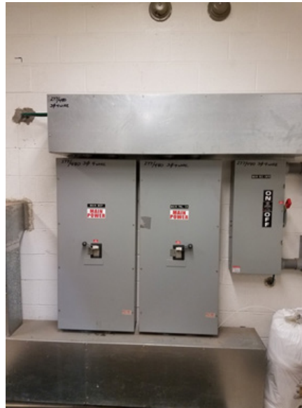
Existing Photo: Building electrical disconnects.
