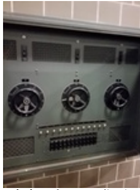
Existing Photo: Auditorium lighting control panel.
