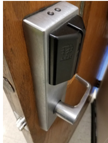
Existing Photo: Card access system, card reader.
